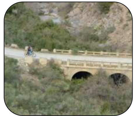
Bridge in Cala Juncols
