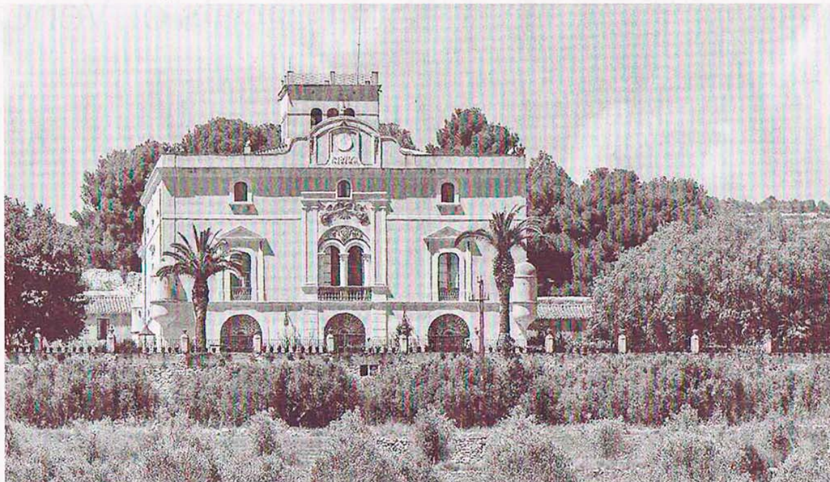
Can Martí, southwest of Barcelona, was influenced by Cuban architecture. The thick-walled defenses, including gun slits, were for protection against bandits, who were active in the late 1800s.
